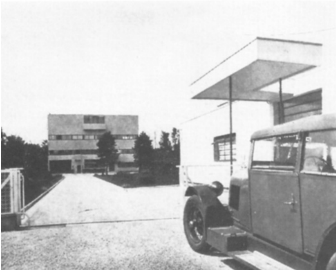
9. Le Corbusier, Villa de Monzie/Stein, Garches, 1927. View of the site threshold. Note the "deep space | collapsed space"—the "outdoor room"—defined by the east-west surface of the villa's north facade and the north-south volume of the gatehouse. (From Oeuvre complète, 1910–1929 , p. 141. Courtesy of Fondation Le Corbusier.)
